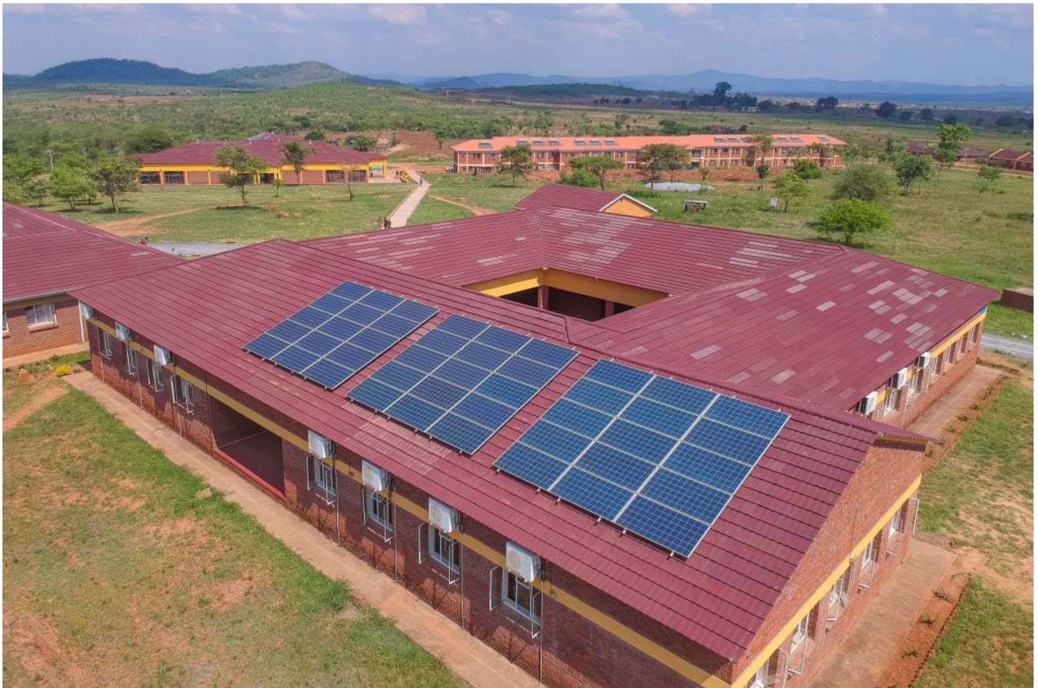
ZEGU ROOF TOPS - Drone shot showing some of the Solar Powered Institution facilities
